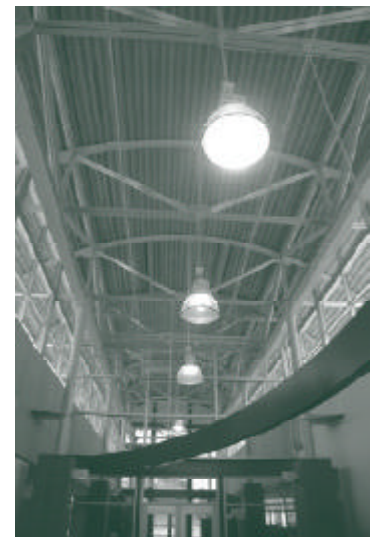
The main entranceway uses curved steel columns and bold colors to create a playful space.
